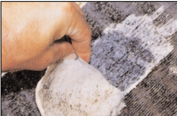
When this coil was removed from service, an interior packed with dirt and grime was revealed, despite hours of cleaning effort.
